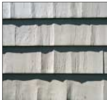
Real wood shakes can warp and split.
